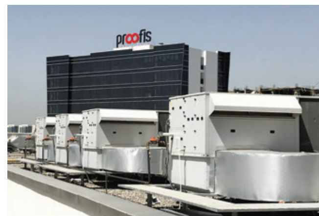
Figure 8: Example retail building installation ©Untes
